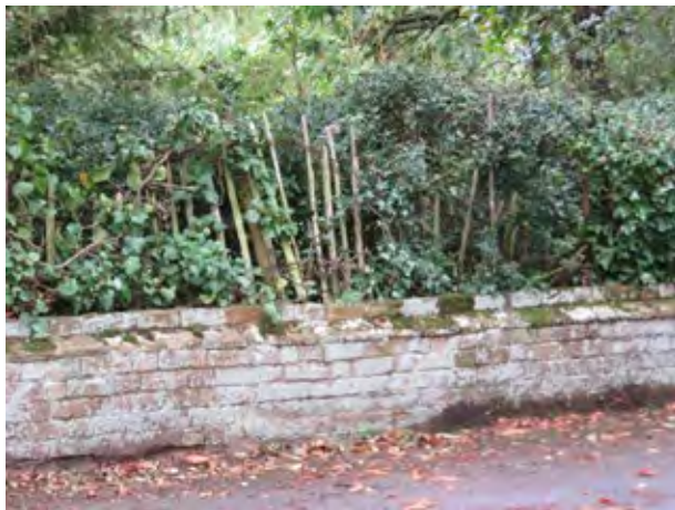
Post and wire replacement fence
