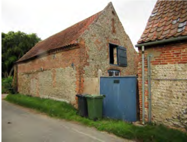
Cedar House barns located at the edge of the garden
