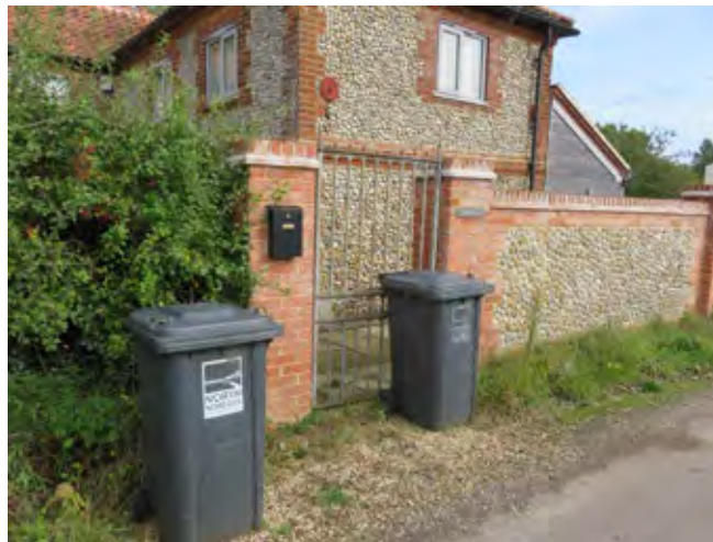
Out of scale new gate piers and wall with letterbox
