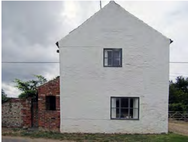
Cottage located north of The Street
