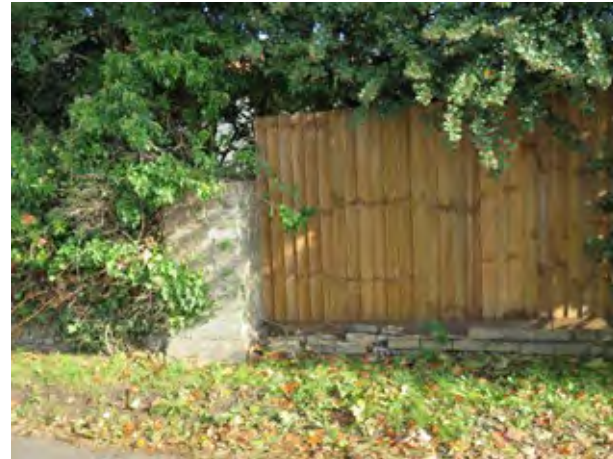
Board fencing has been used to replace a historic wall
