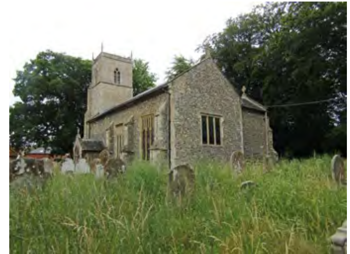
View of east and south elevation of the church from the churchyard
