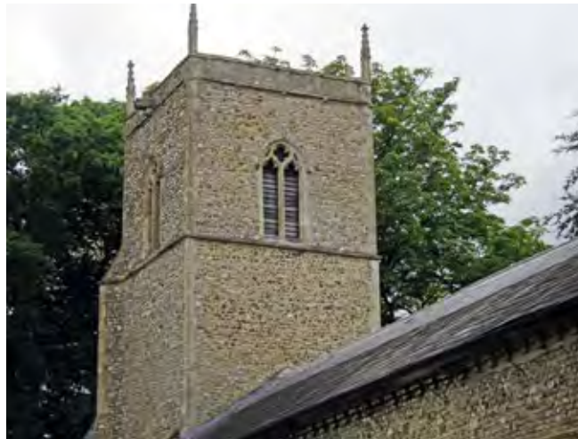
Detailed view of the church tower
