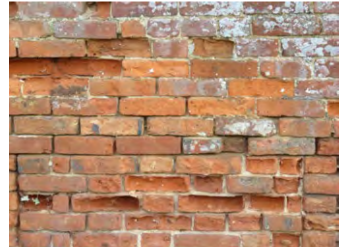
Eroding brickwork
