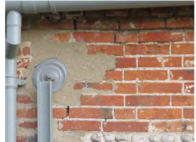
Cementitious repointing to brickwork
