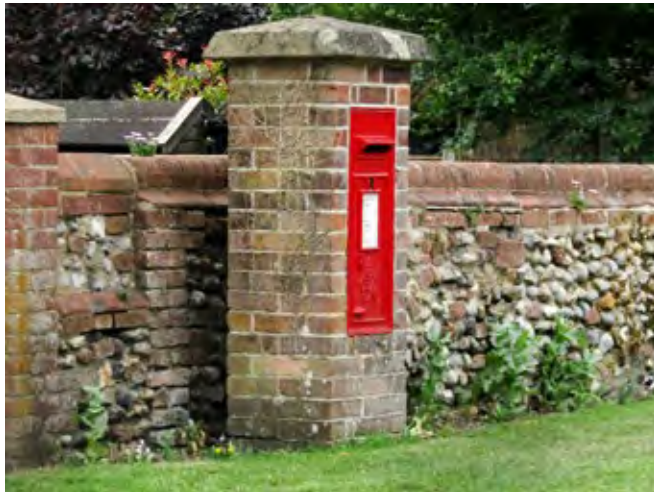
Wall post box on the east side of The Street near to the phone box
