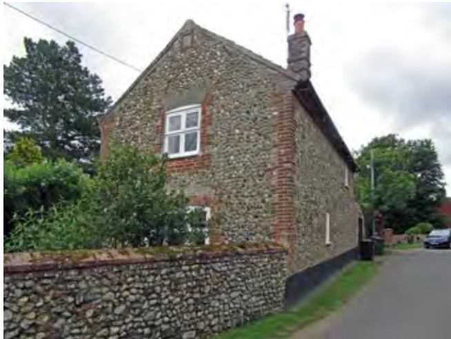
Cobble flint and red brick Stonewall Cottage on The Street
