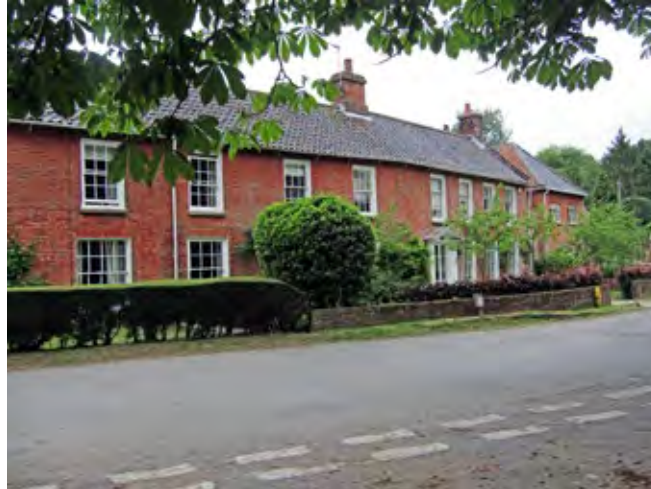
Small hedge and walling fronting the late-eighteenth century houses west of the Green
