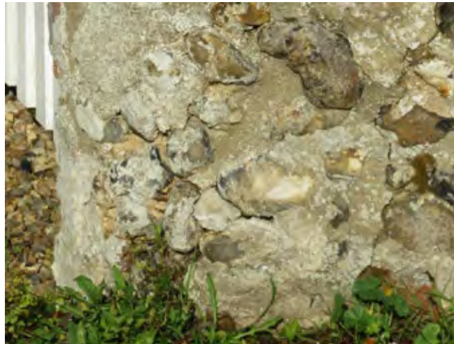
Cementitious pointing to a flint wall
