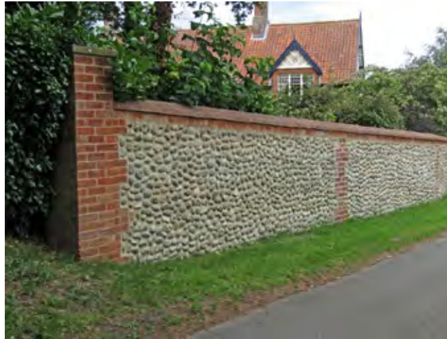
New wall at The Grange north of Stody Road
