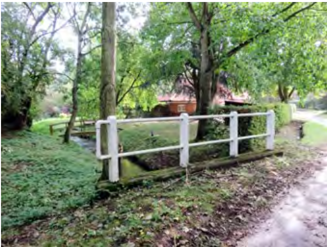
Bridge railing separating public right of way from tributary of the River Glaven
