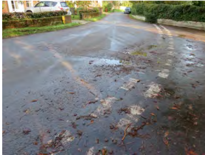
Patched road surface
