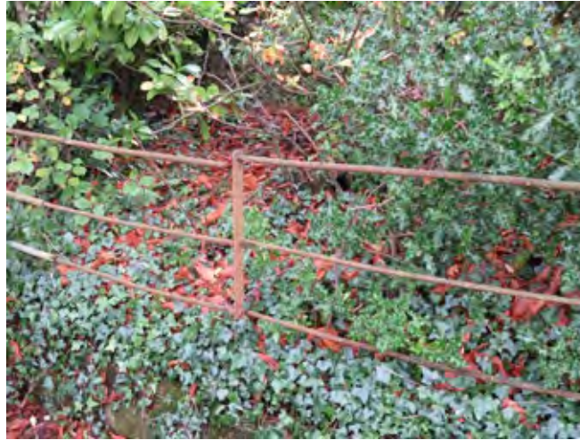
Metal railing to the churchyard
